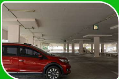
COVERED CAR PARKING
